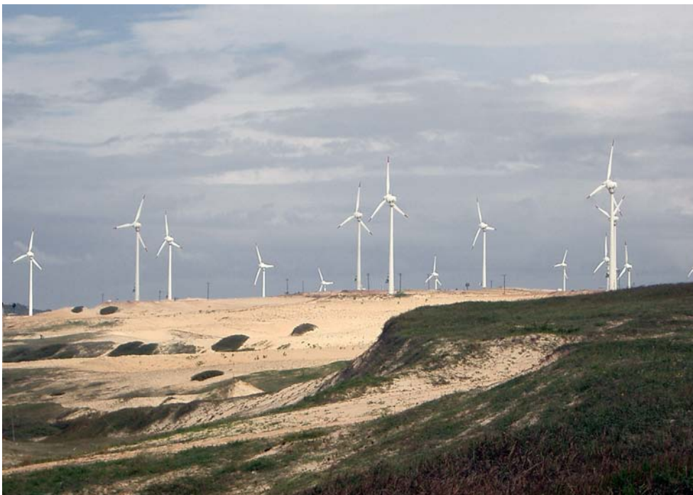
Figure 1: Brazil's largest wind park: Prainha (30 km from Fortaleza, in the Northeast of Brazil) with 20 wind turbines of 500 kW each, representing about 40% of the country's wind power capacity presently installed.
