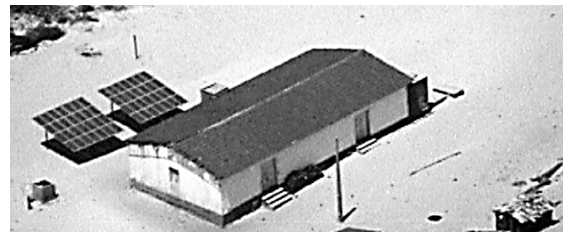
Figure 4: Installation site at the coast of Apiques, close to Baleia, NE-Brazil: building of the PV-powered ice manufacture and the two PV panels (2.5 kW p each).
